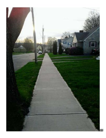
Sidewalks on Holly Street all have smooth, firm surfaces and are free of hazards or obstacles. However, some parts of the sidewalk have a cross slope greater than the 2% (1.1 degree) maximum recommended by the CHII and none of them met the required width of five feet across.
